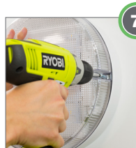
Use captive screws to screw the diffuser into place
