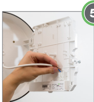
Safely connect supply
